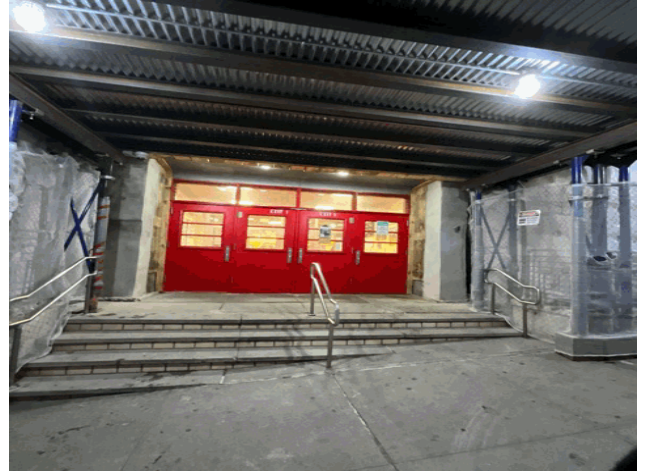
Facade A - West 130th Street
