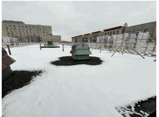
Roof 1 - Southeast View
