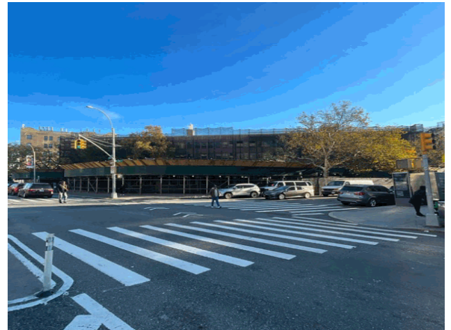
Corner of St. Nicholas Avenue and West 168th Street - Northeast View
