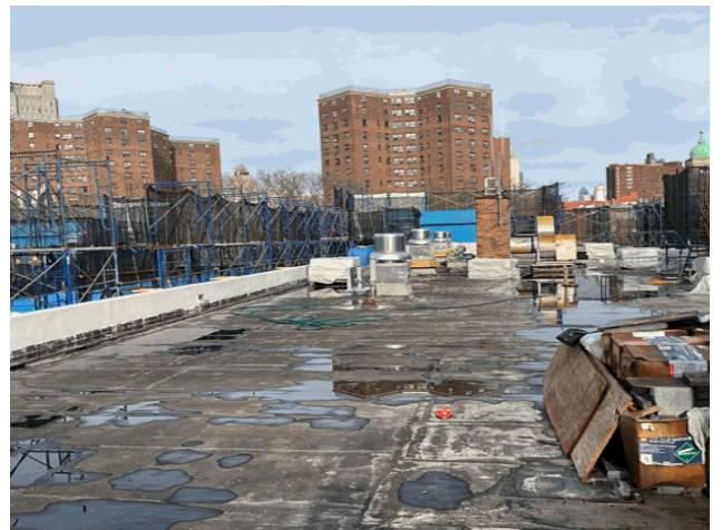
Roof 1 - North View
