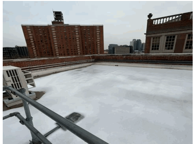
Roof 4 - East View
