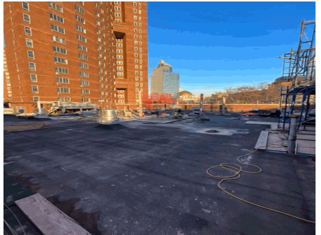
Roof 1 - Northwest View
