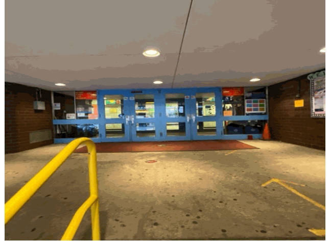
Facade A - Division Street
