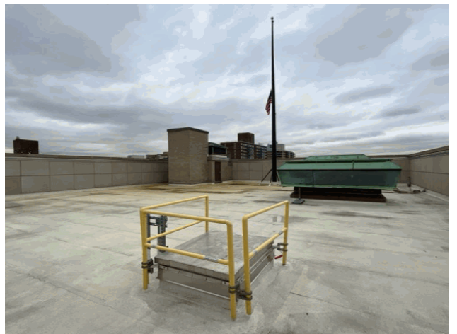
Roof 1 - North View
