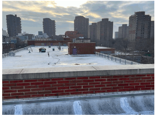
Roof 8 - Southeast View
