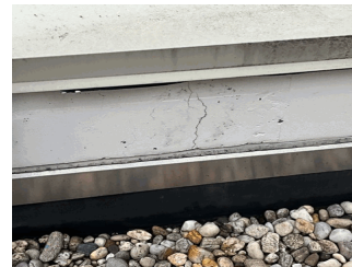
Roof 1 - Facade B
