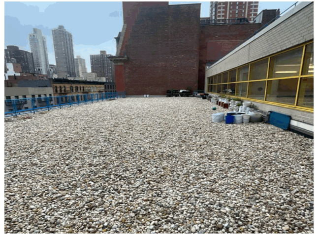
Roof 2 - West View
