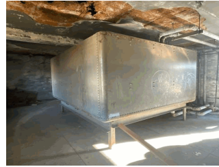
Roof Tank Room
