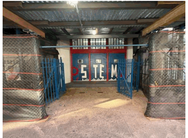
Facade A - West 113th Street
