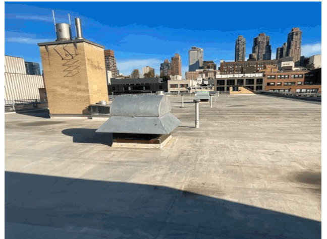
Roof 1 - Northeast View
