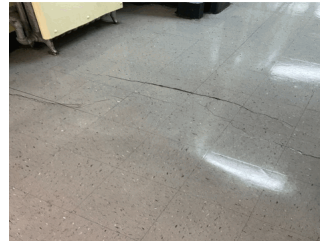
Corridor near Room 506
