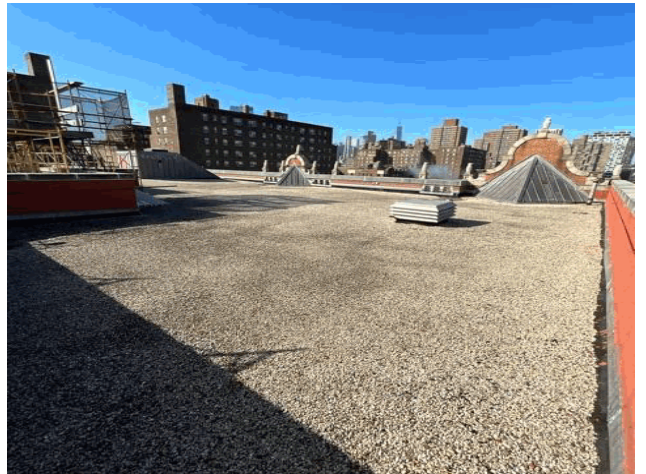
Roof 1 - West View
