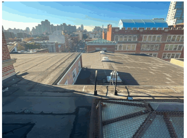
Roof 2 - Southwest View
