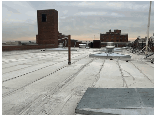
Roof 1 - East View
