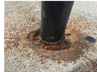
Facade E - HC Ramp
