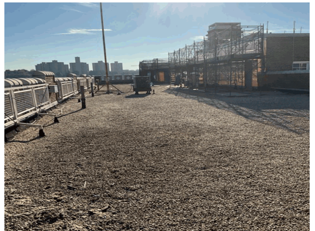
Roof 1 - Southeast View
