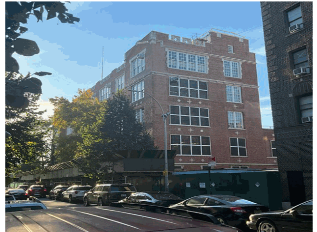
West 212th Street - Southeast View
