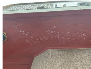
Above Main Entrance
