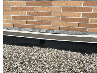
Facade A near Bulkhead BH2
