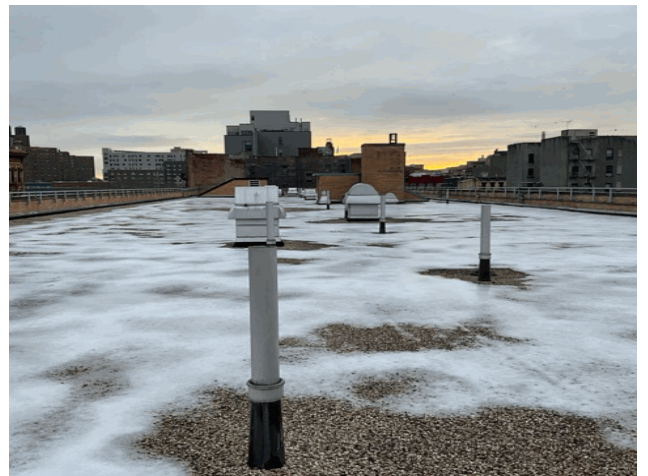
Roof 1 - Southeast View
