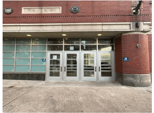
Facade A - Warren Street
