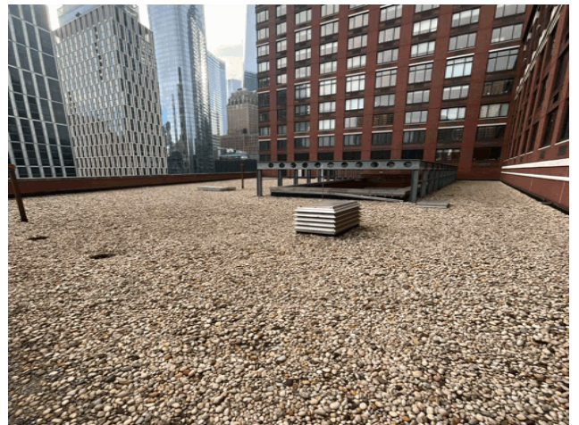
Roof 1 - South View
