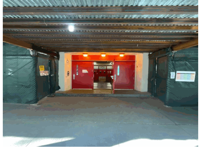
Facade A - West 78th Street
