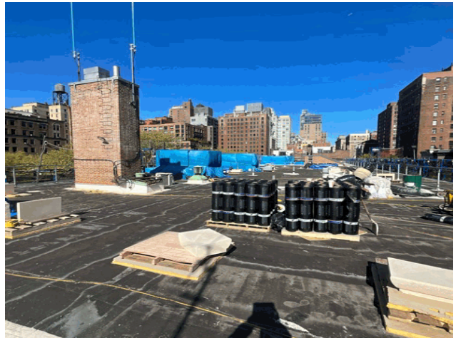
Roof 1 - Northwest View
