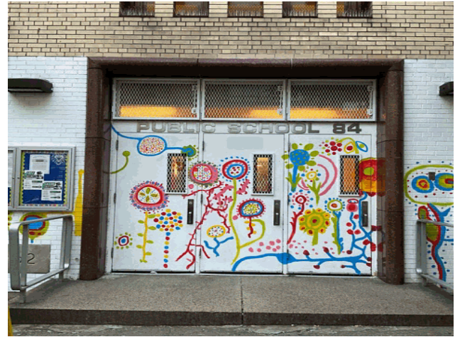
Facade A - West 92nd Street
