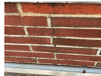
Roof 1 - Facade E
