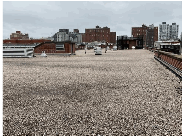
Roof 1 - Northwest View
