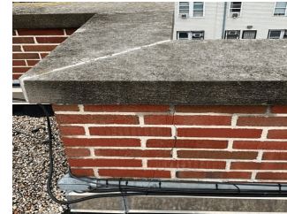
Roof 1 - Facade E
