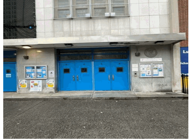
Facade A - West 109th Street
