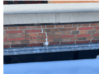
Facade G at Roof 1
