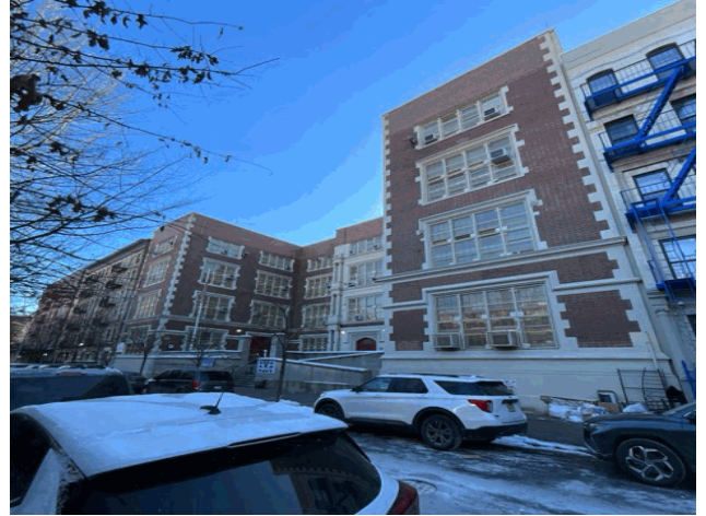
Facade A - West 120th Street
