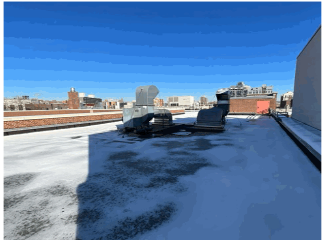
Roof 2 - North View
