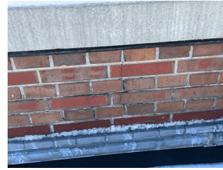
Facade G at Roof 1
