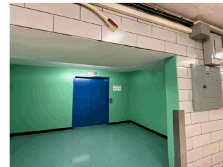
Elevator Lobby - 3rd Floor
