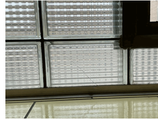
Facade G - 2nd Floor Corridor
