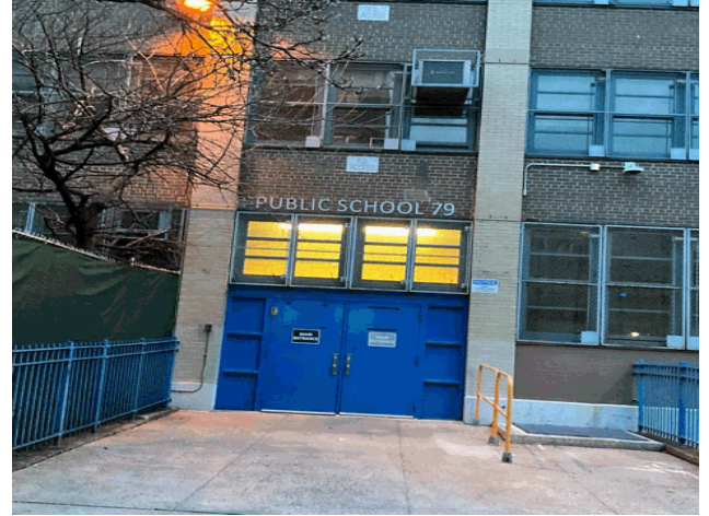
Facade A - East 120th Street
