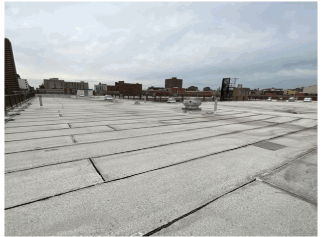
Roof 1 - West View
