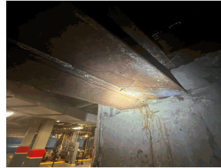
Ash Hoist Vault
