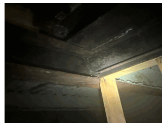
Ash Hoist Vault
