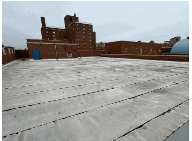
Roof 3 - Northeast View
