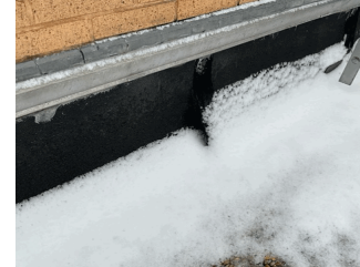
Facade E at Roof 4
