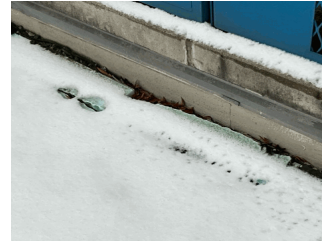
Roof 2 at Facade B
