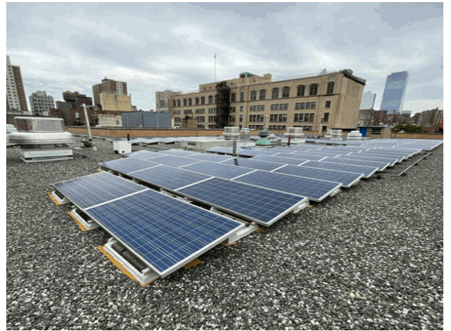
Roof 1 - North View
