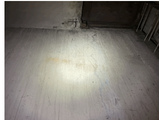
Ash Hoist Vault
