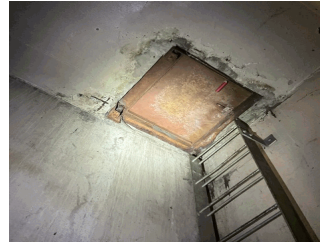
Ash Hoist Vault
