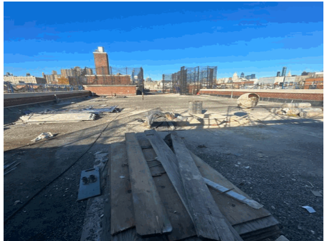
Roof 1 - West View
