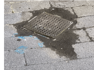
Roof 2 - Plaza Deck near Exit 4
