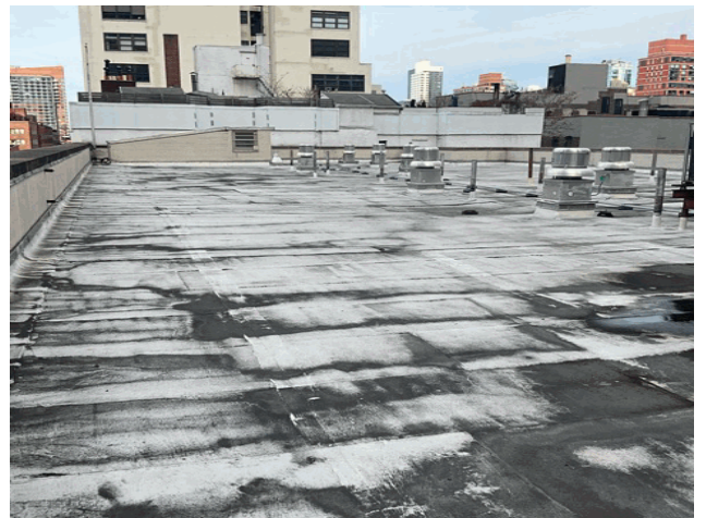
Roof 1 - Northwest View
