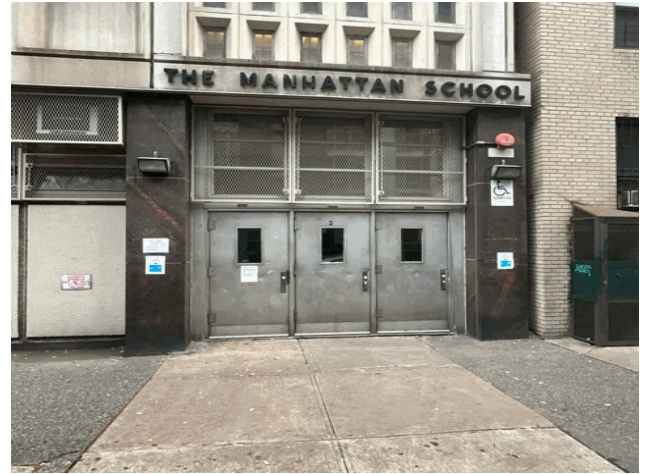
Facade A - West 52nd Street
