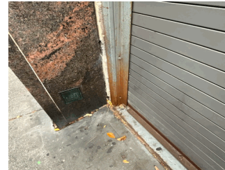
Facade A - Auto Shop Exit
