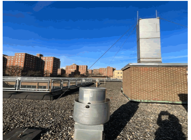
Roof 1 - West View
