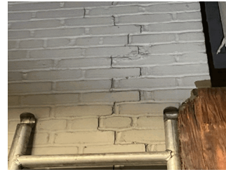
Mechanical Equipment Room 201
