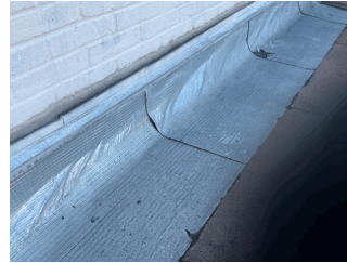
Roof 1 - Facade E
