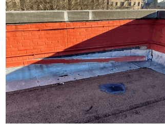
Roof 1 - Facade A
