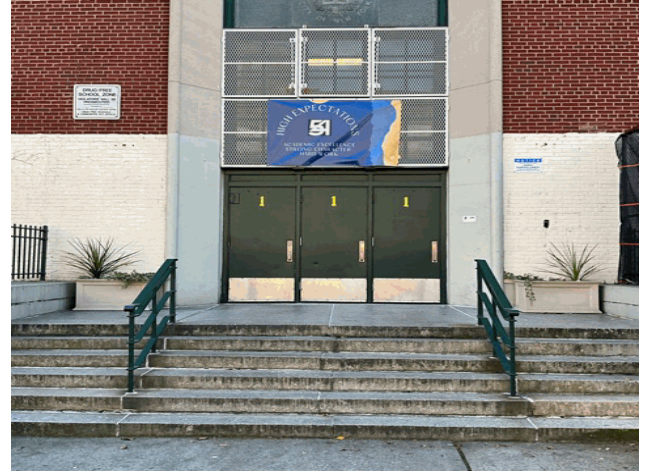
Facade A - West 108th Street
