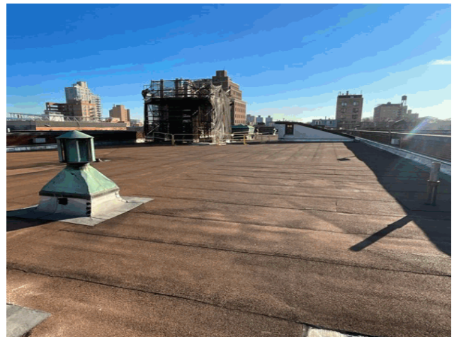
Roof 1 - East View
