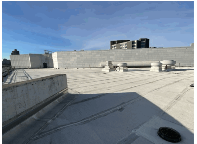
Roof 3 - West View
