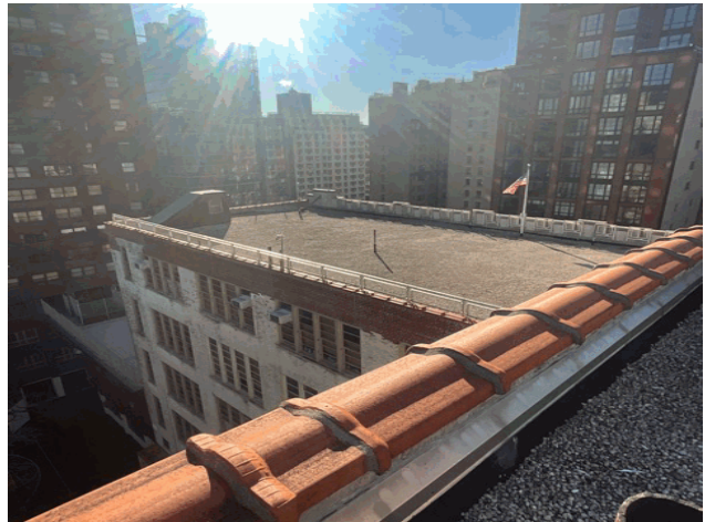
Roof 3 - South View
