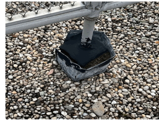
Roof 1 - Facade A
