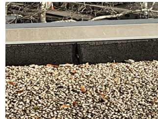
Roof 1 - Facade K
