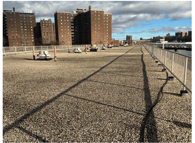
Roof 1 - Northeast View
