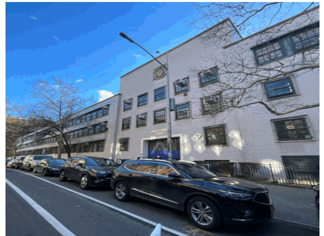
West 77th Street - South View
