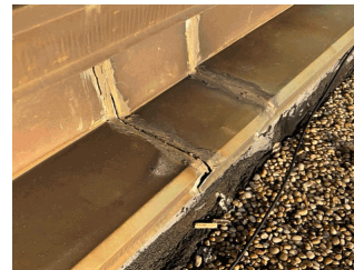
Penthouse (right of door to Roof 1)
