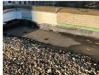
Roof 3 at Facade G
