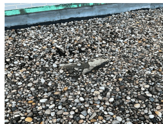
Roof 3 near Bulkhead BH2
