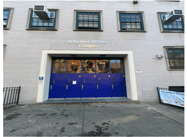
Facade A - West 77th Street
