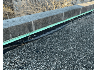
Facade D on Roof 4
