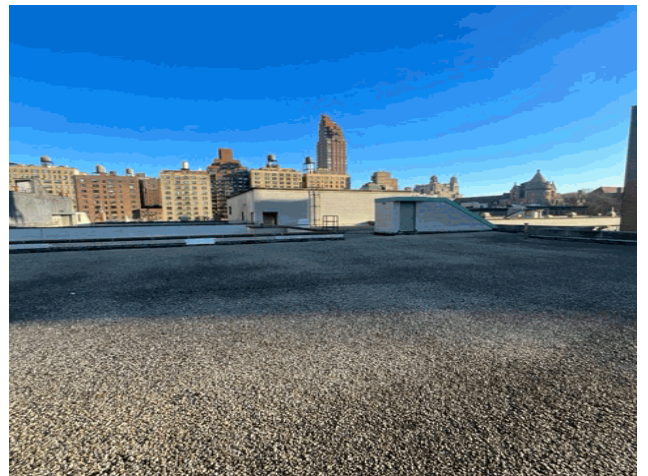
Roof 4 - Northeast View
