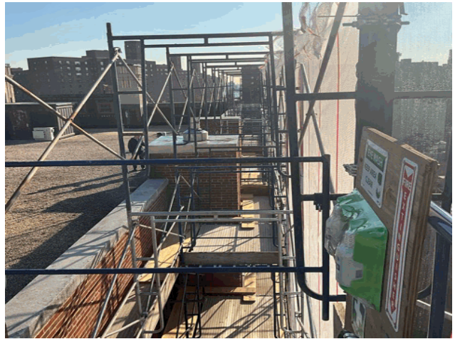
Roof 1 - Southeast View
