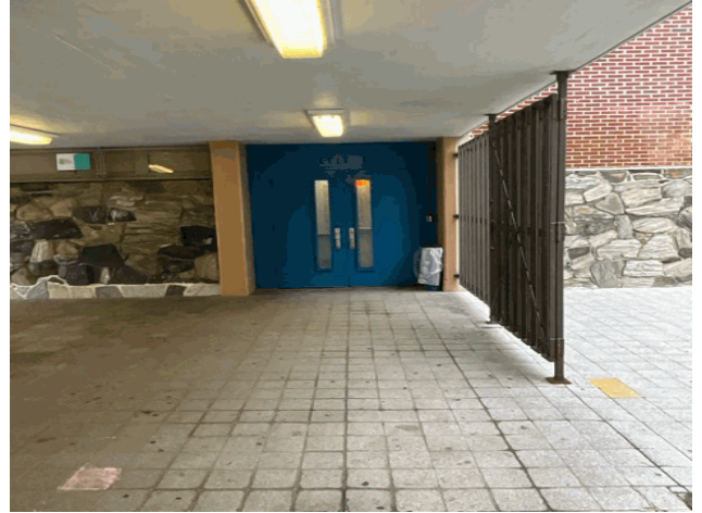
Facade A - Morningside Drive
