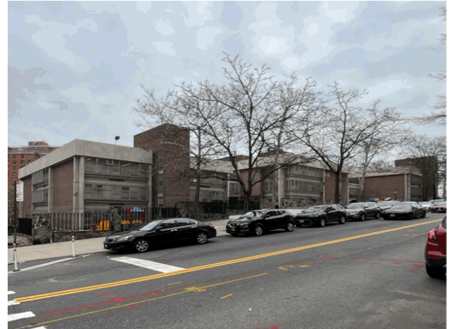
Corner of Morningside Drive and Amsterdam Avenue - East View
