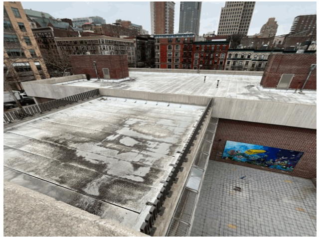
Roof 4 - East View
