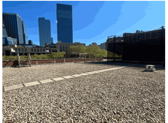
Roof 1 - Northwest View
