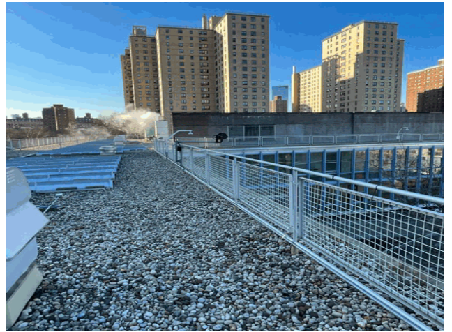
Roof 1 - Southwest View
