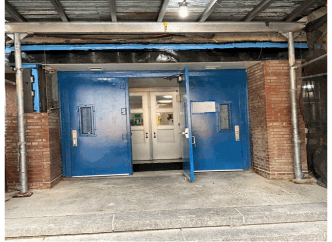
Facade A - Essex Street
