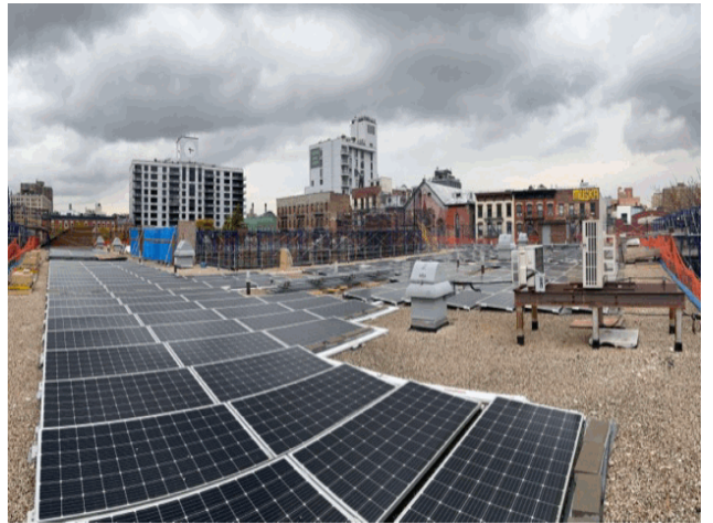
Roof 1 - East View
