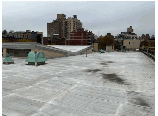
Roof 1 - West View
