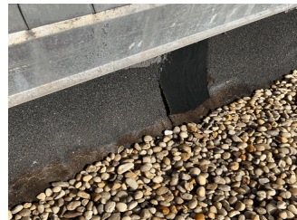
Roof 1 - Facade A
