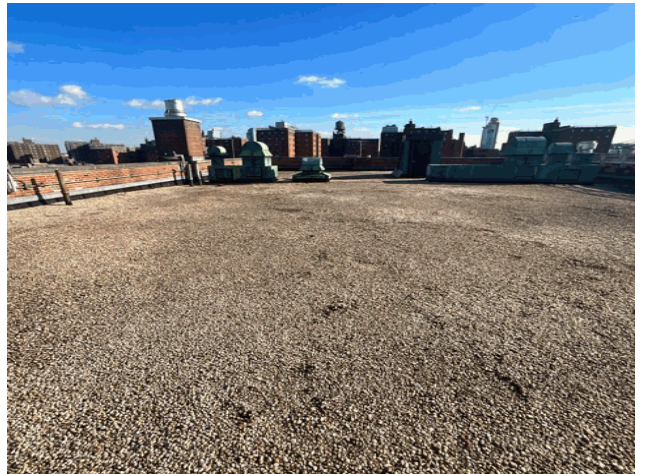
Roof 1 - East View
