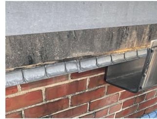
Roof 1 - Facade C
