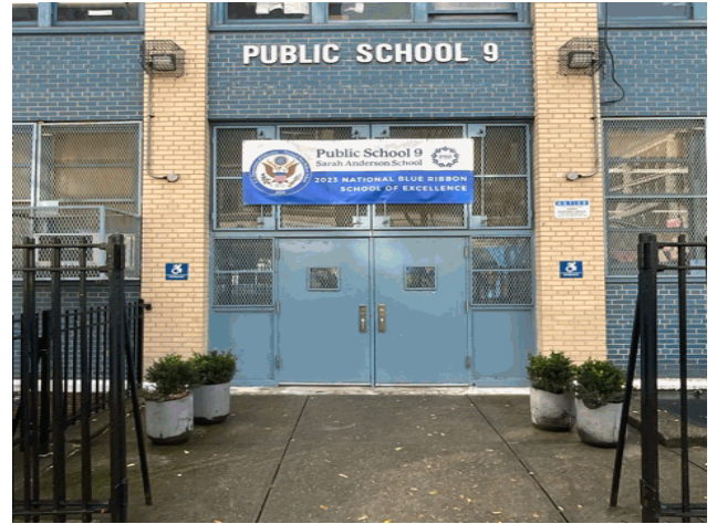
Facade A - West 84th Street
