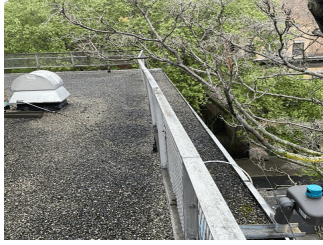
Roof 1 at Facade D
