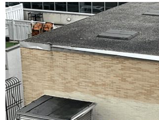
Roof 3 at Facade E1
