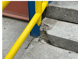
West Exit on Facade H
