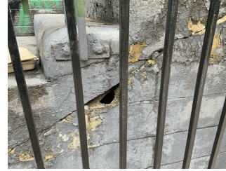
Gymnasium exit at Facade H
