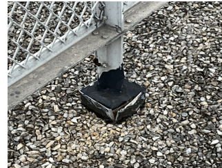
Roof 1 at Facade D
