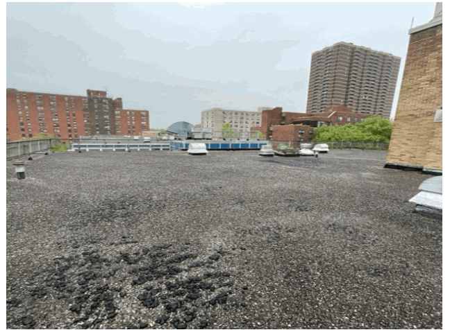
Roof 1 - Northwest View
