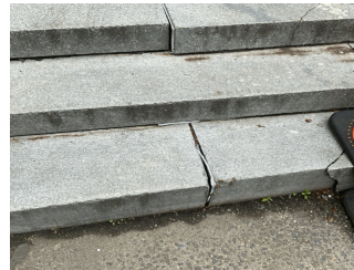
Exit 4 (near loading dock)
