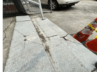
Entrance near Loading Dock
