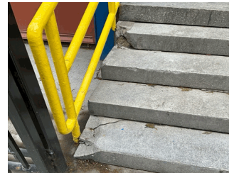
West Exit on Facade H
