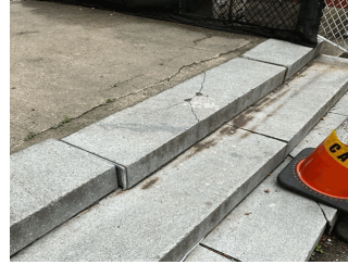
Facade D at Exit 4
