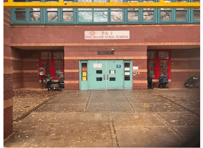
Facade A - Harlem River Drive
