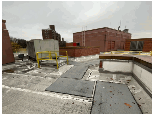
Roof 2 - North View
