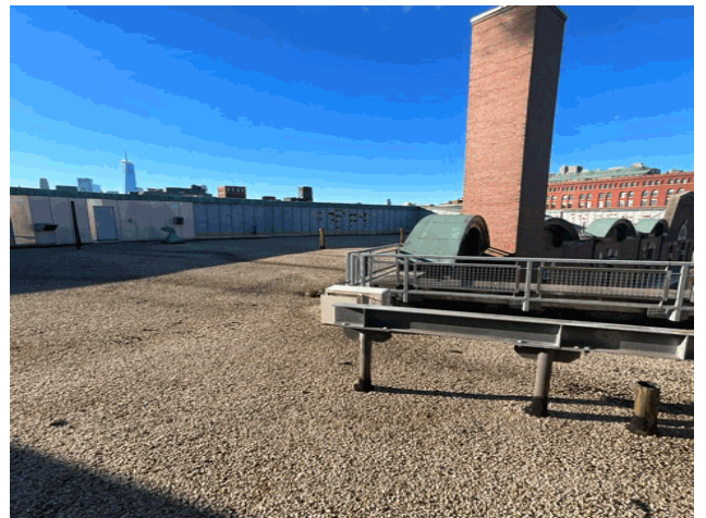
Roof 1 - West View
