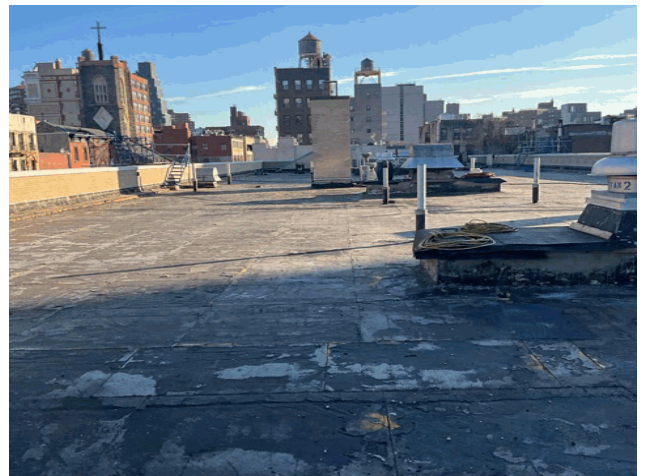
Roof 1 - East View
