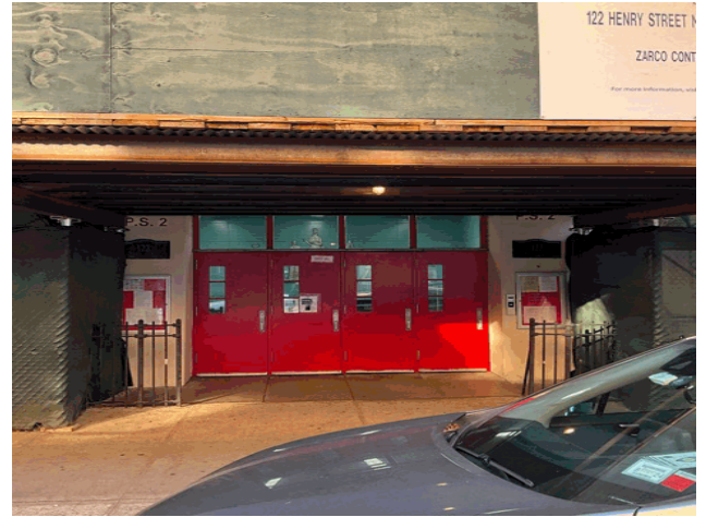
Facade A - Henry Street
