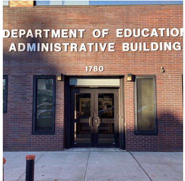
Facade A - Ocean Avenue
