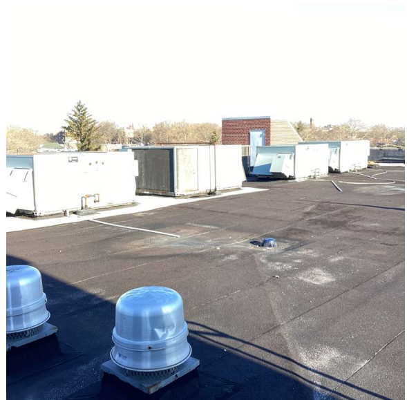
Roof 1 - North View
