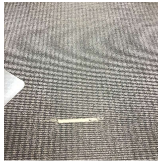
2nd Floor cubicle area
