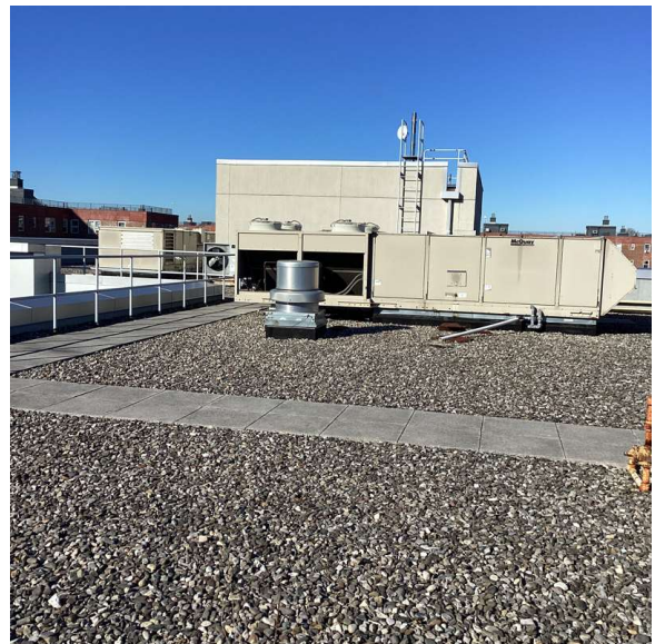
Roof 1 - Northwest View
