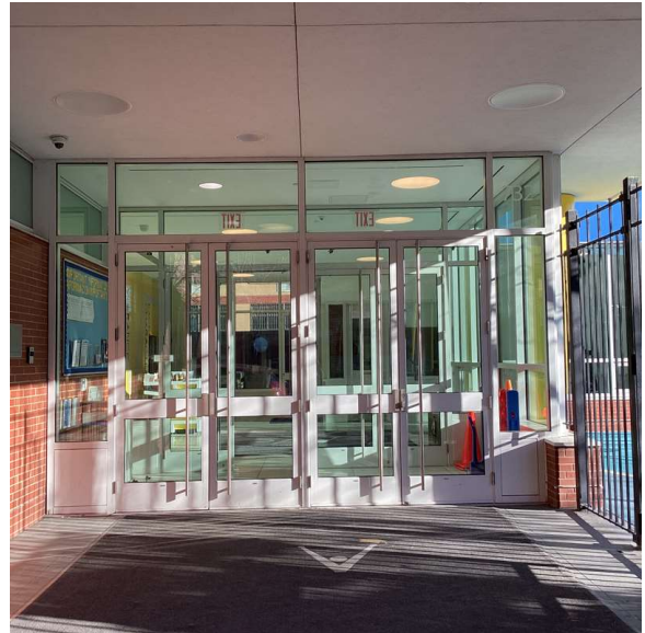
Facade A - Mill Street
