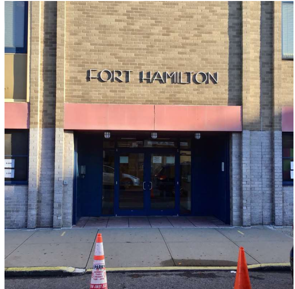
Facade A - 89th Street
