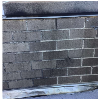
Roof 3 - Facade B
