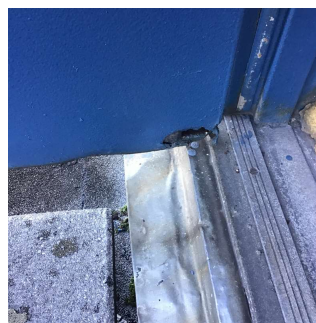
Facade C - Exit to Roof 3
