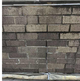
Roof 3 - Facade C
