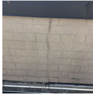
Roof 2 - Facade A
