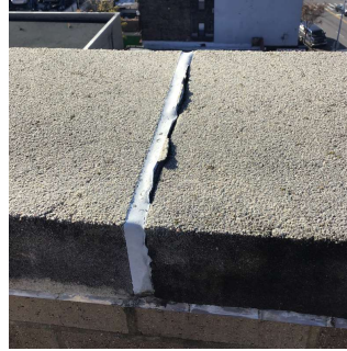
Roof 1 - Facade A
