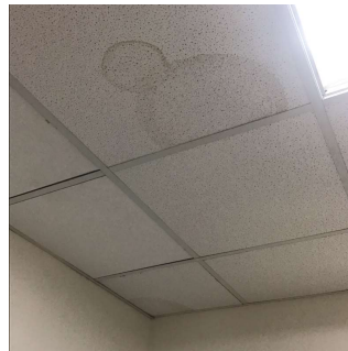
Roof 3 - Room 116 No violations recorded.
