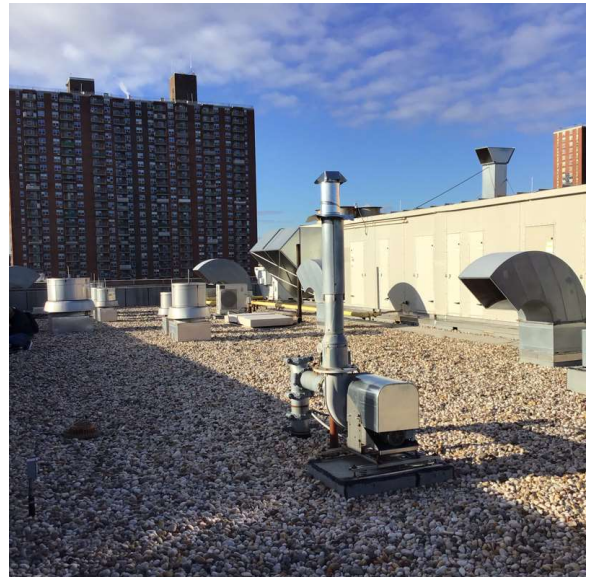
Roof 1 - North View
