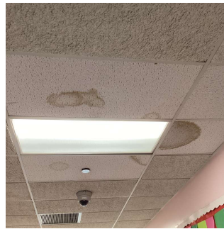
Corridor near Room 404
