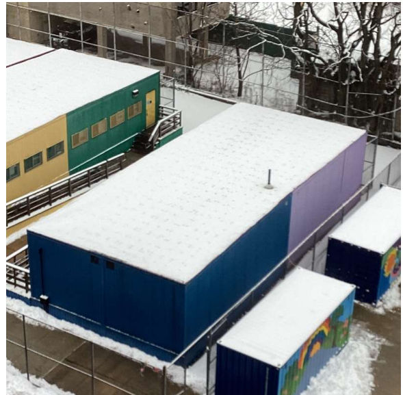
Roof 1 - Northeast View
