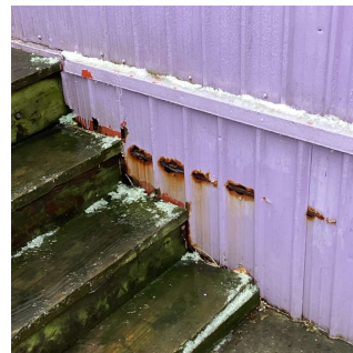
Facade A - Unit T2
