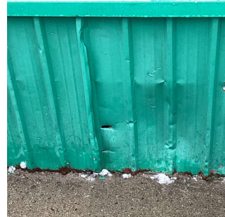
Facade E - Unit T3
