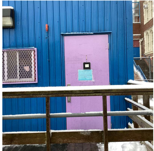
Facade A - T1
